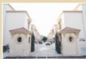
Shalimar Homes Lawrence Terrace, Ashok Marg
