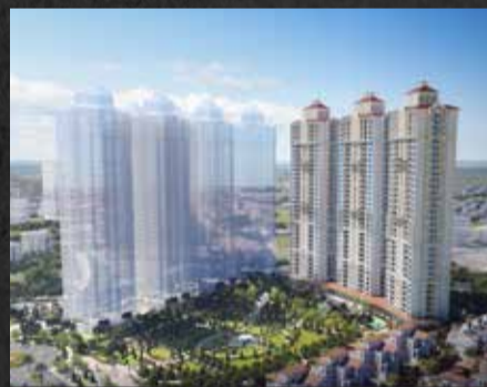
Valencia Towers Gomti Nagar Extension UPRERAPRJ496663
